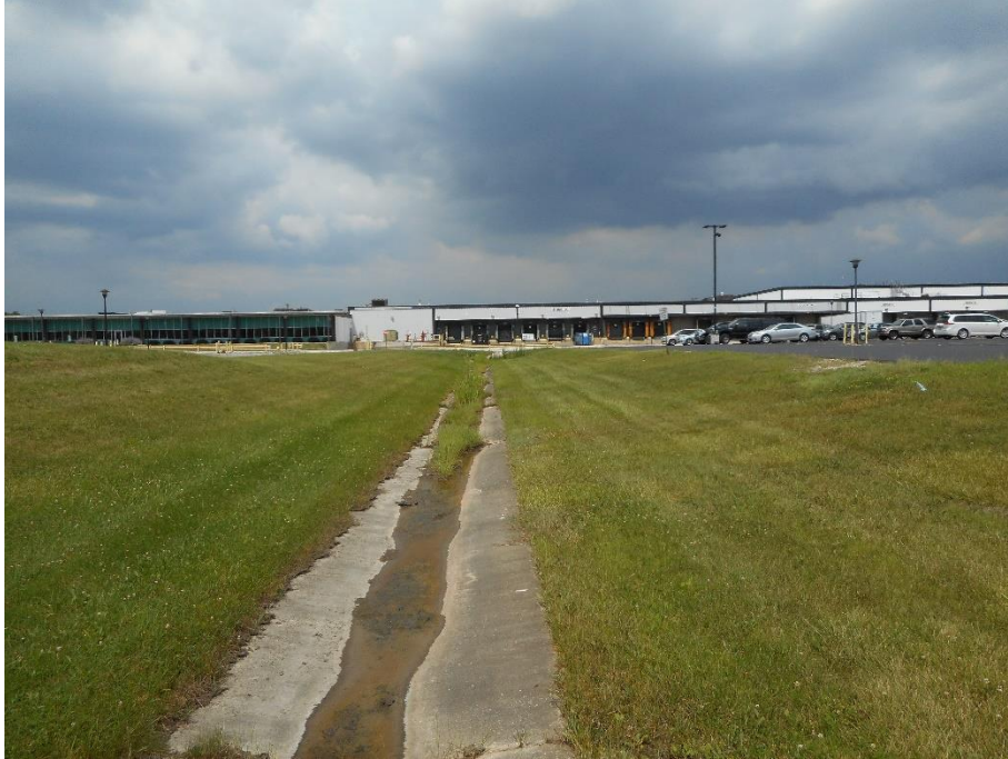
PHOTOGRAPH 9: View looking to the north at the drainage swale that runs along the eastern portion of the site.
