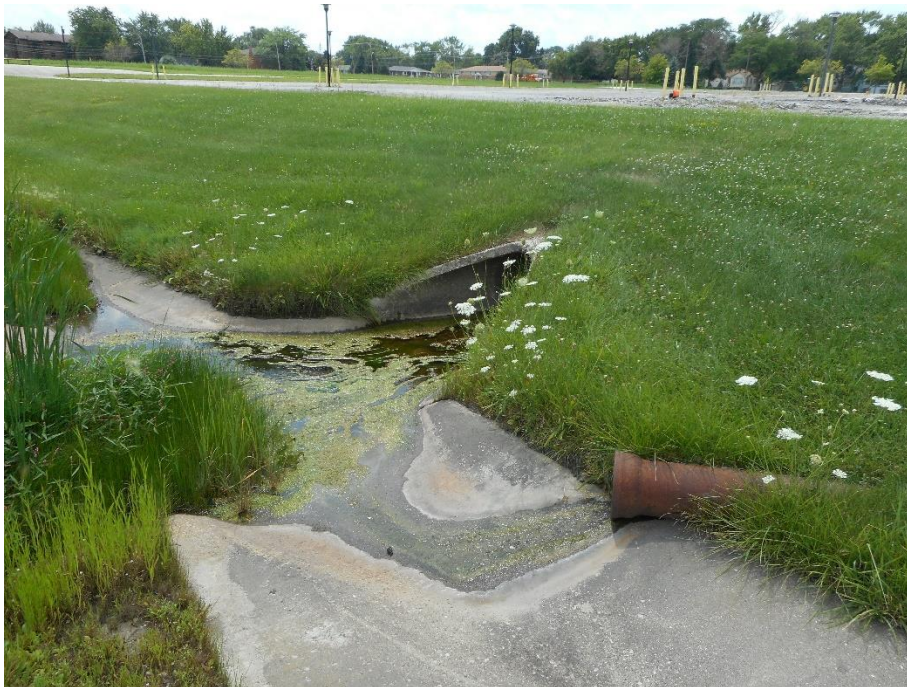
PHOTOGRAPH 8: View looking to the south at the drainage swale from the northeast corner of the site.
